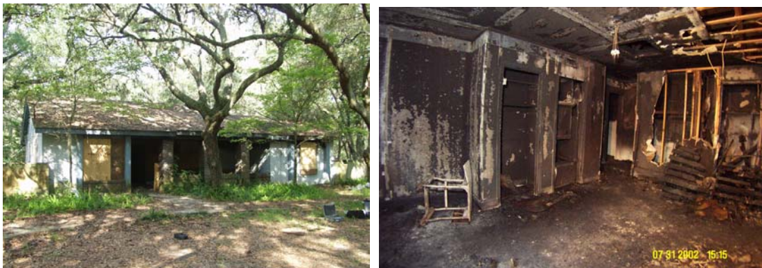
Figure 1. Outside of acquired structure and interior of fire room.
